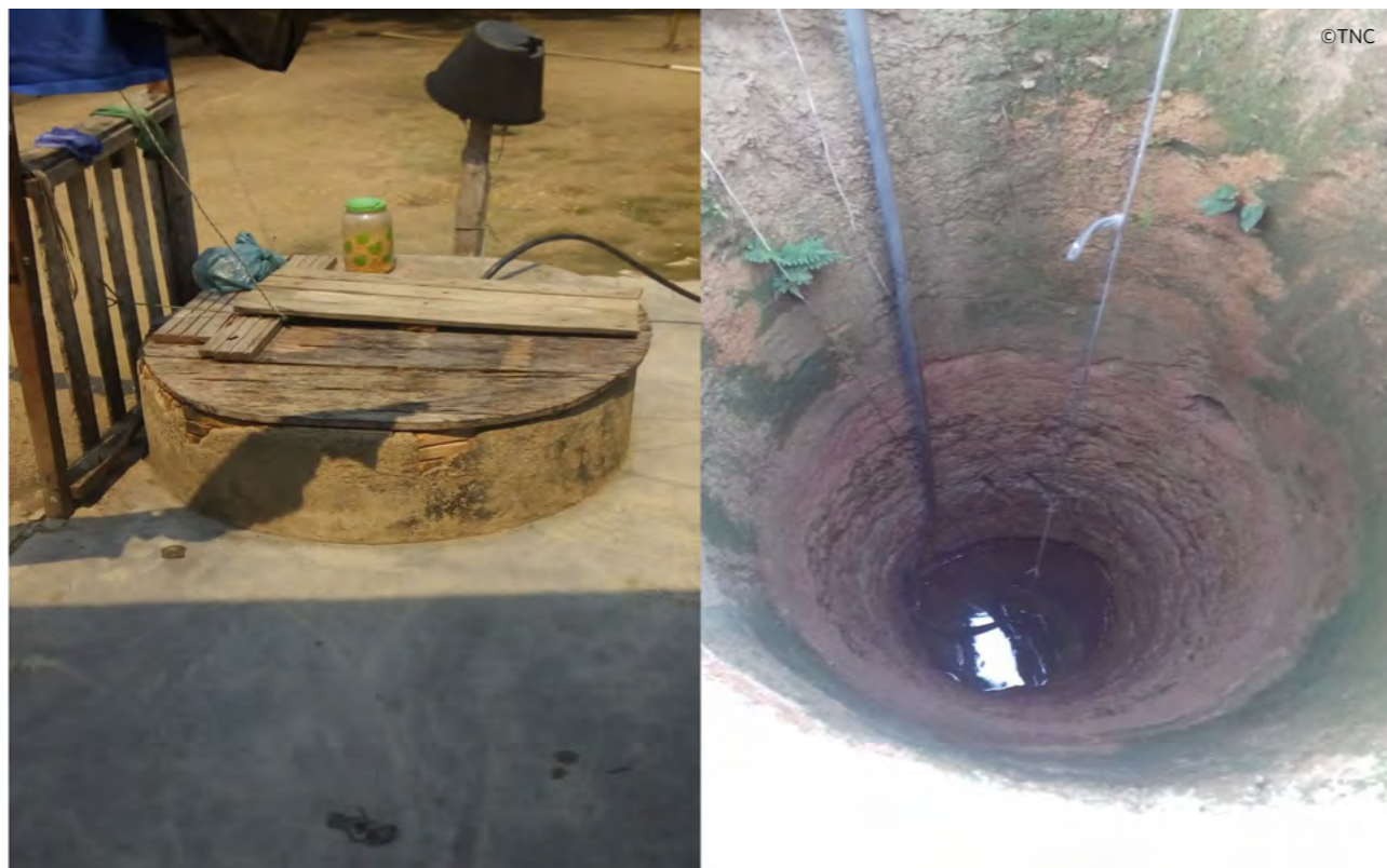
Figure 6 - Amazon wells and pumping system. Source: Pimental community association collection.
